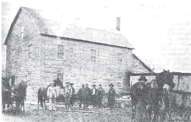
Dicks Mill, date unknown, Adolph Dick stands on the left in miller's cap. He is covered with flour dust.
